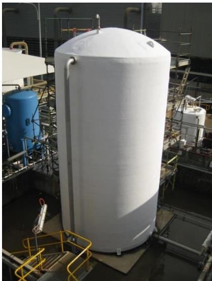
Figure 1 – A typical FRP Process Tank
