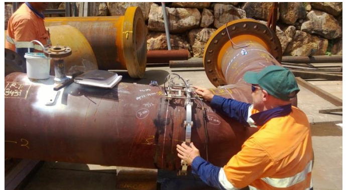
Figure 1 - Large Diameter Heavy Wall Scanning using PAUT.
