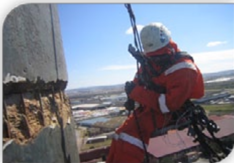
Rope access to remediation site of a stack
