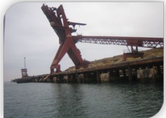
Overall view of wharf structure
