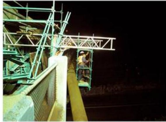
**Figure 2 Night work assembling the hanging scaffold**
